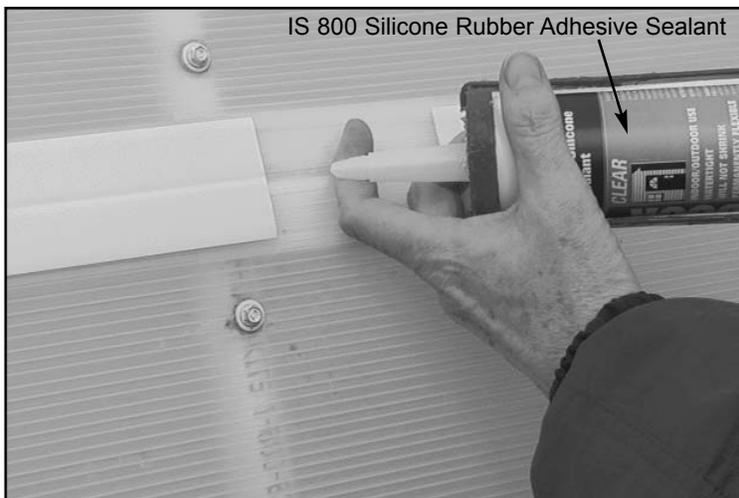
2. From the outside of the greenhouse, insert about a nickel-size gob of silicone caulking into the area between the H-Channel pieces.
